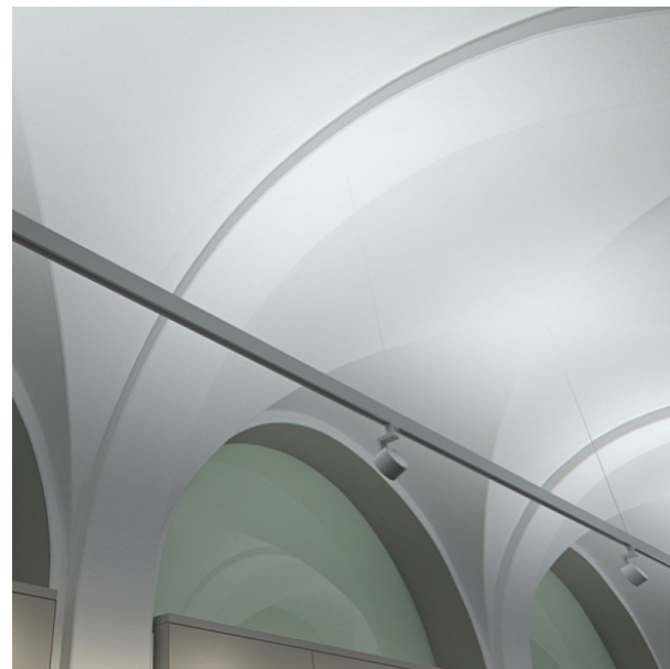
(Erco 'Hi-trac track and light structure)
